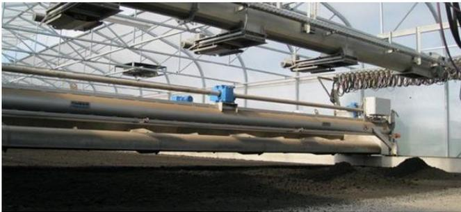
Atmospheric control is automatically controlled via fans mounted at the “dry” end of the greenhouse. Louvers are provided at the opposite “wet” end. The ventilation of the greenhouse is controlled based on air temperature and humidity in the greenhouse and in the environment. Additional fans are installed under the roof and blow warm air vertically onto the Biosolids layer.
